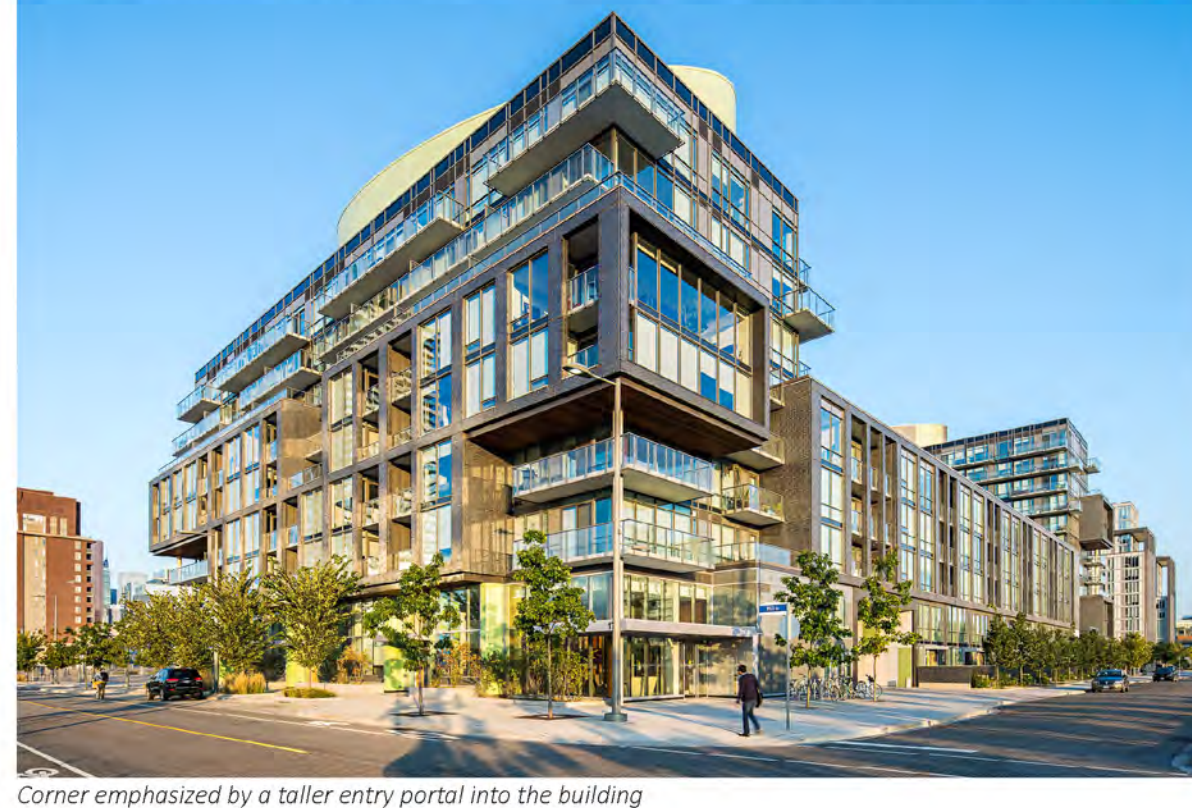
Corner emphasized by a taller entry portal into the building.
