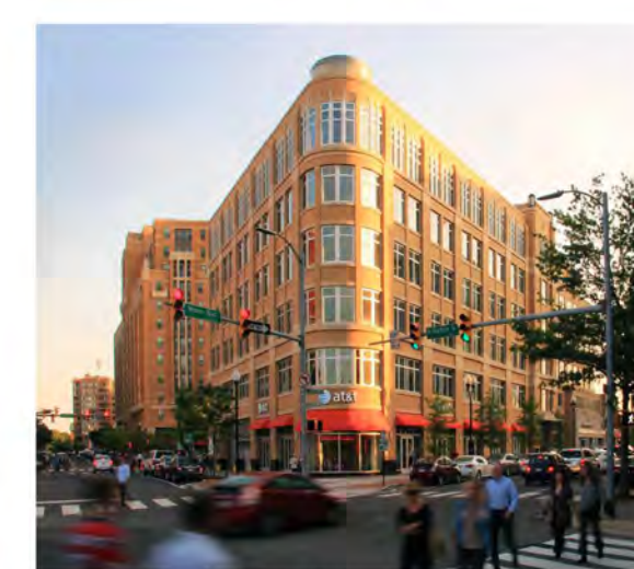
A rounded architectural treatment at the corner.
