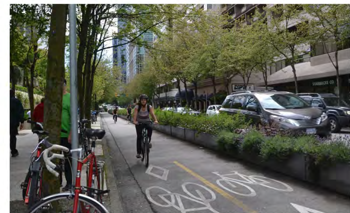
A separated bike lane buffered by landscape provides a safe and efficient route for cyclists.
