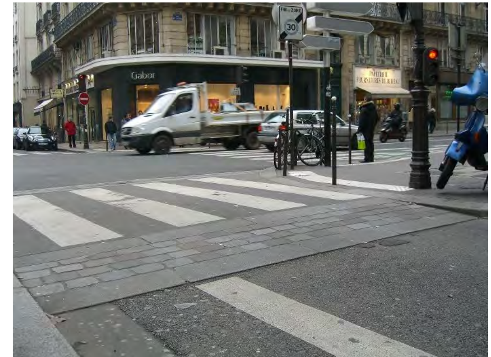
A raised crossing at sidewalk-level across a low-speed, low-volume street. Photo: Vladimir Zlokazov
