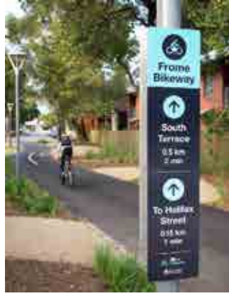
Frome Street Bikeway; Adelaide, Australia - Wayfinding Sign (Source: urbanandpublic.com)
