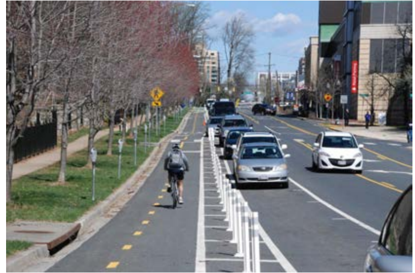
Woodglen Drive Two-Way Separated Bike Lanes (2014) (Source: MCDOT)
